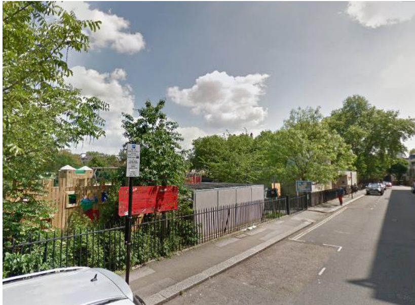
Photo 2 – View of existing fence to be replicated (left side of photo) and entrance to site (right side of photo)
