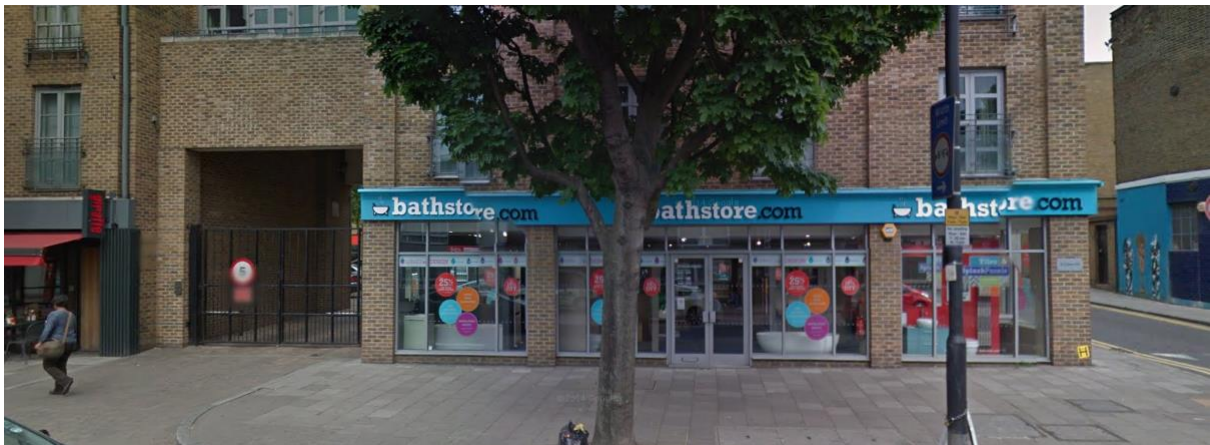
Image 3. Photo of the application site as seen from Essex Road
