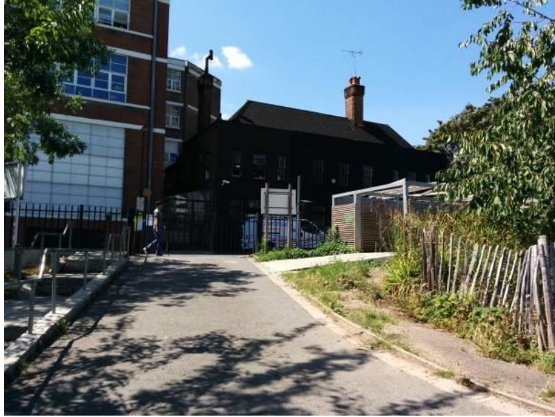
Photo 1 – Location of proposed fence across existing entrance
