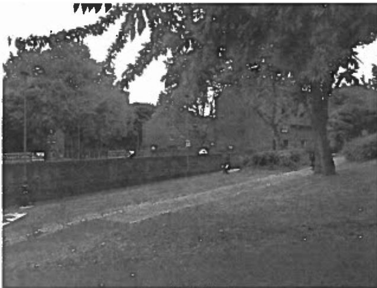
Image 6: View from North
