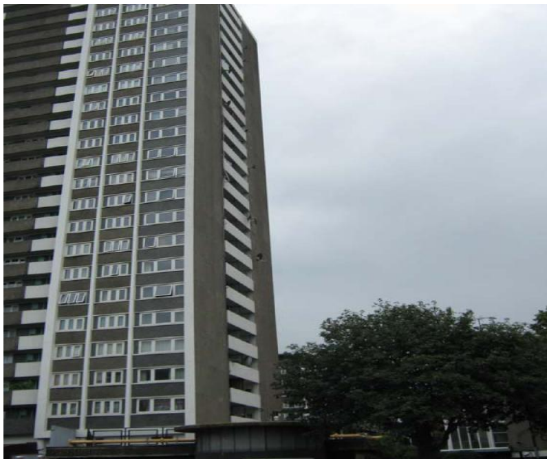
Image 2: Distant view front elevation (facing west) of Michael Cliffe House from Skinner Street
