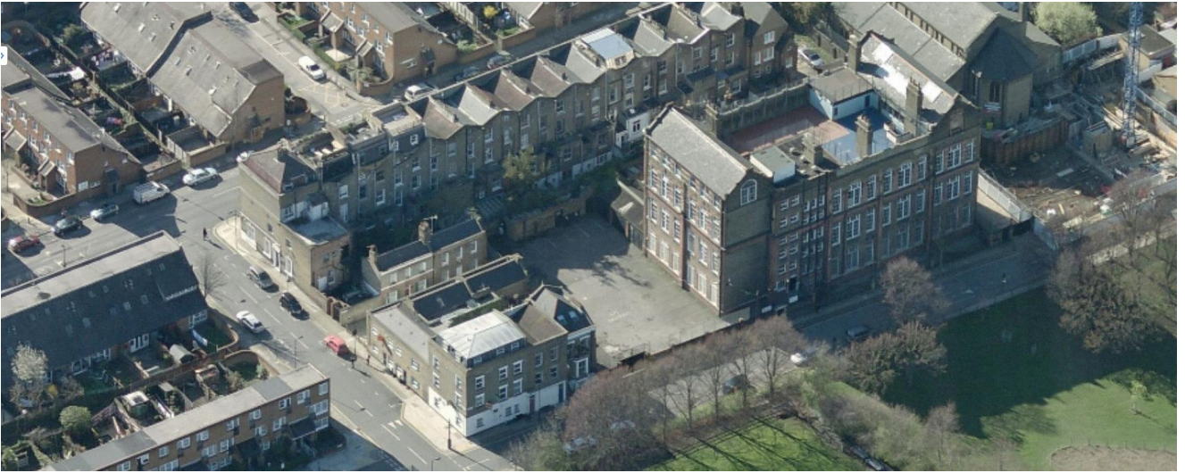
Image 1: Aerial view of street elevation
